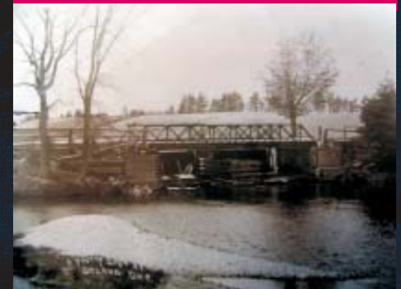
The mill bridge was made of timber and was part of the dam that ensured there was adequate water available to run the water wheel.
