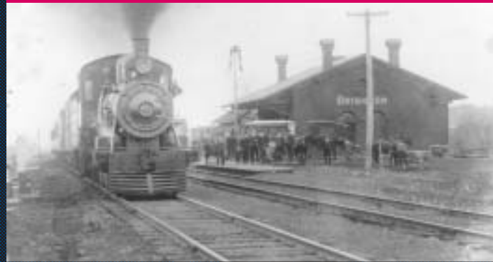
The Brighton train station promoted the development of industry and agriculture in the local area.
